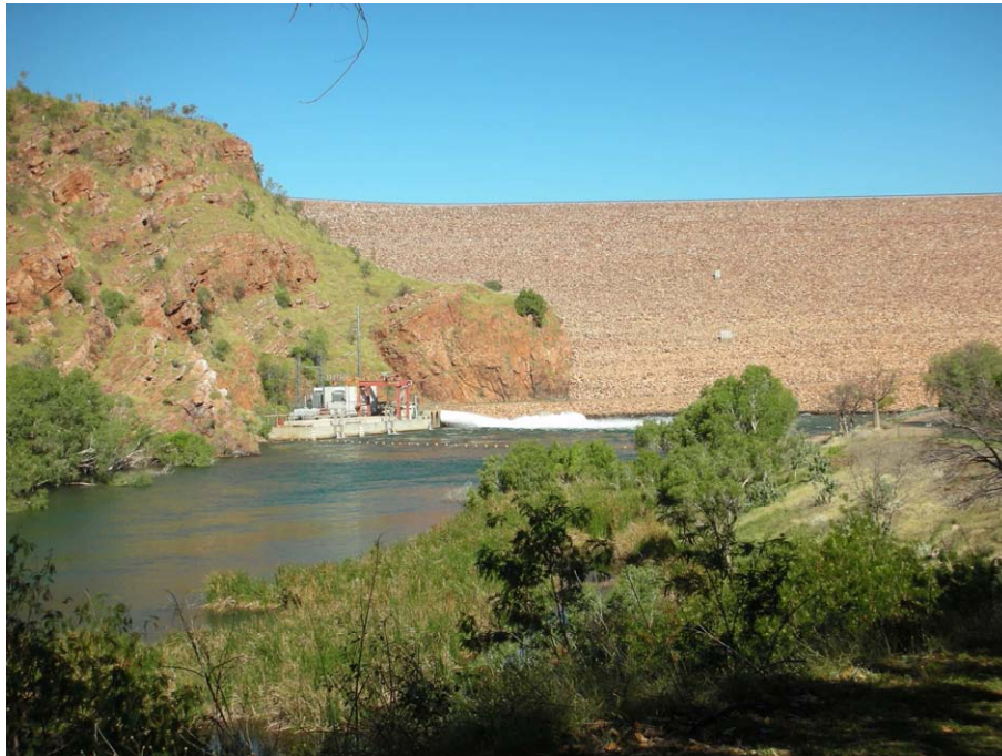
Plate 3: Dam wall at Lake Argyle with hydroelectric power station at its base
